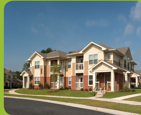
FIGURE 7: REDEVELOPMENT SAMPLE PHOTO
