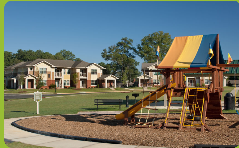
FIGURE 5: REDEVELOPMENT SAMPLE PHOTO
