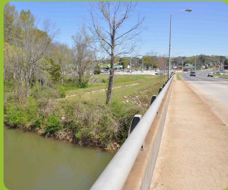
10TH STREET ADJACENT TO THE CHATTAHOOCHEE RIVER REPRESENTS A STRATEGIC LOCATION AND IS A PRIME OPPORTUNITY FOR A FUTURE CATALYST PROJECT
