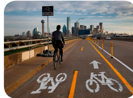
10th Street bridge traffic volumes support a reduction in the total number of vehicular travel lanes.
